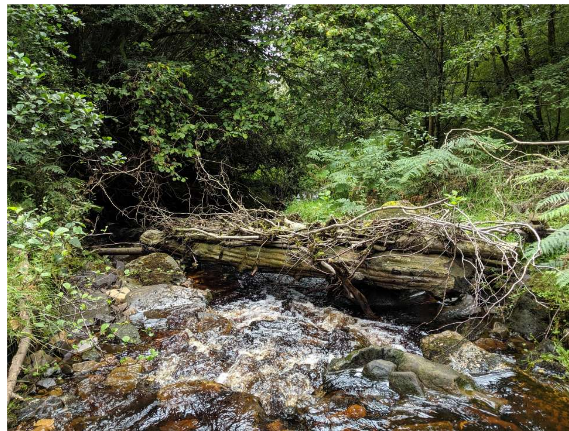
Figure 1: Failed leaky dam, North Yorkshire
