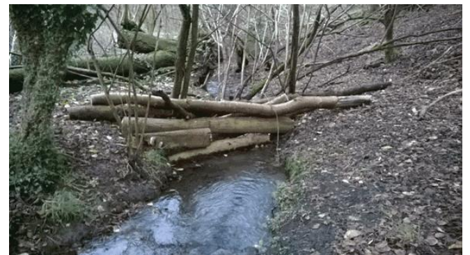
Woody debris dam, Stroud Rural Sustainable Drainage Systems scheme. Credit: Stroud.gov.uk
