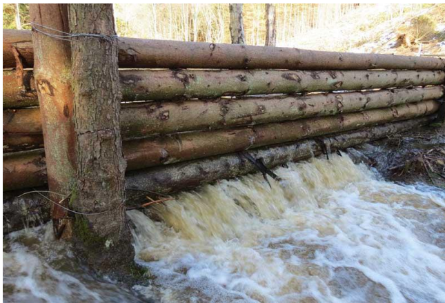
Timber bund at Pickering. Credit: Institution of Civil Engineers
