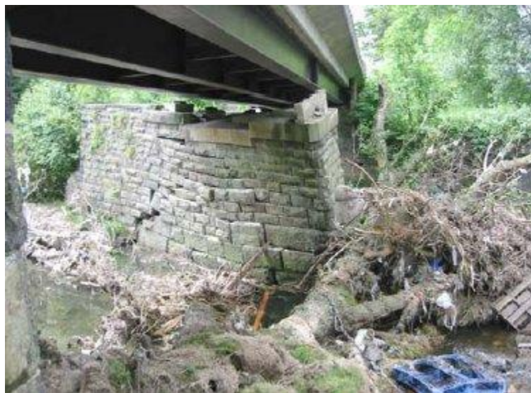
Figure 2. Lower Ashenbottom Viaduct, Lancashire, UK; partial collapse of central pier after the flood of June 2002 where scour is thought to have been exacerbated by debris collection on the central pier (photograph courtesy of Bury Metropolitan Council Engineering Services)
