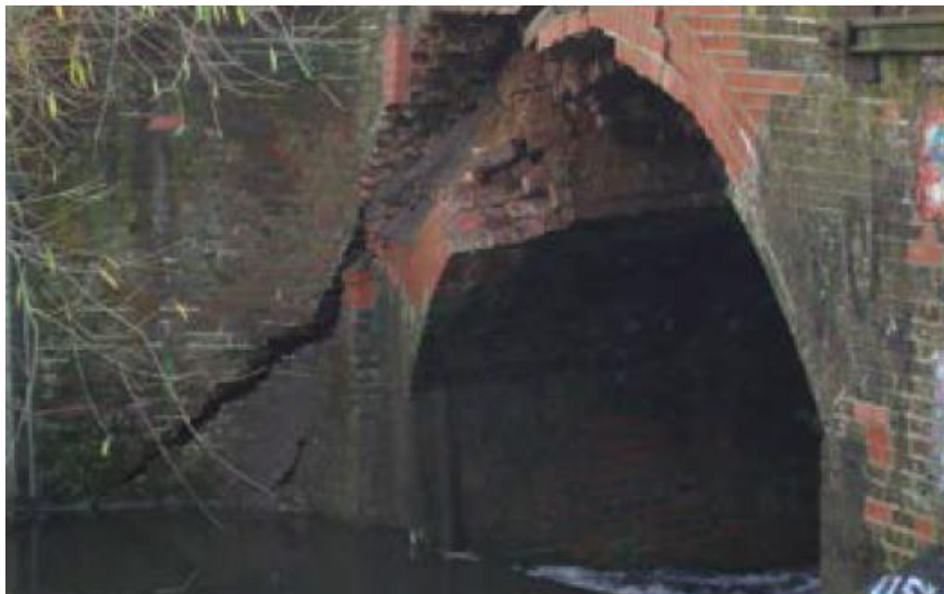
Figure 1. Railway bridge collapse caused by scour at Feltham on the River Crane, West London, in November 2009
