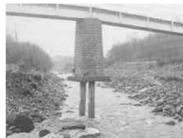
General or natural scour resulting in exposure of bridge foundations.
