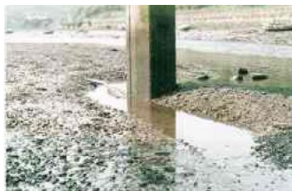
Bridge pier is 1.6m wide and 4m long. Direction of flow is from left to right
